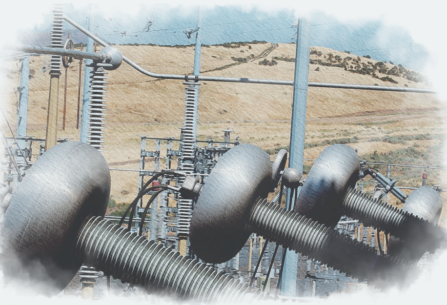
Wall bushings with corona rings draw electricity to and from the transformers into the valves, in The Dalles, Ore., in this file photo.
