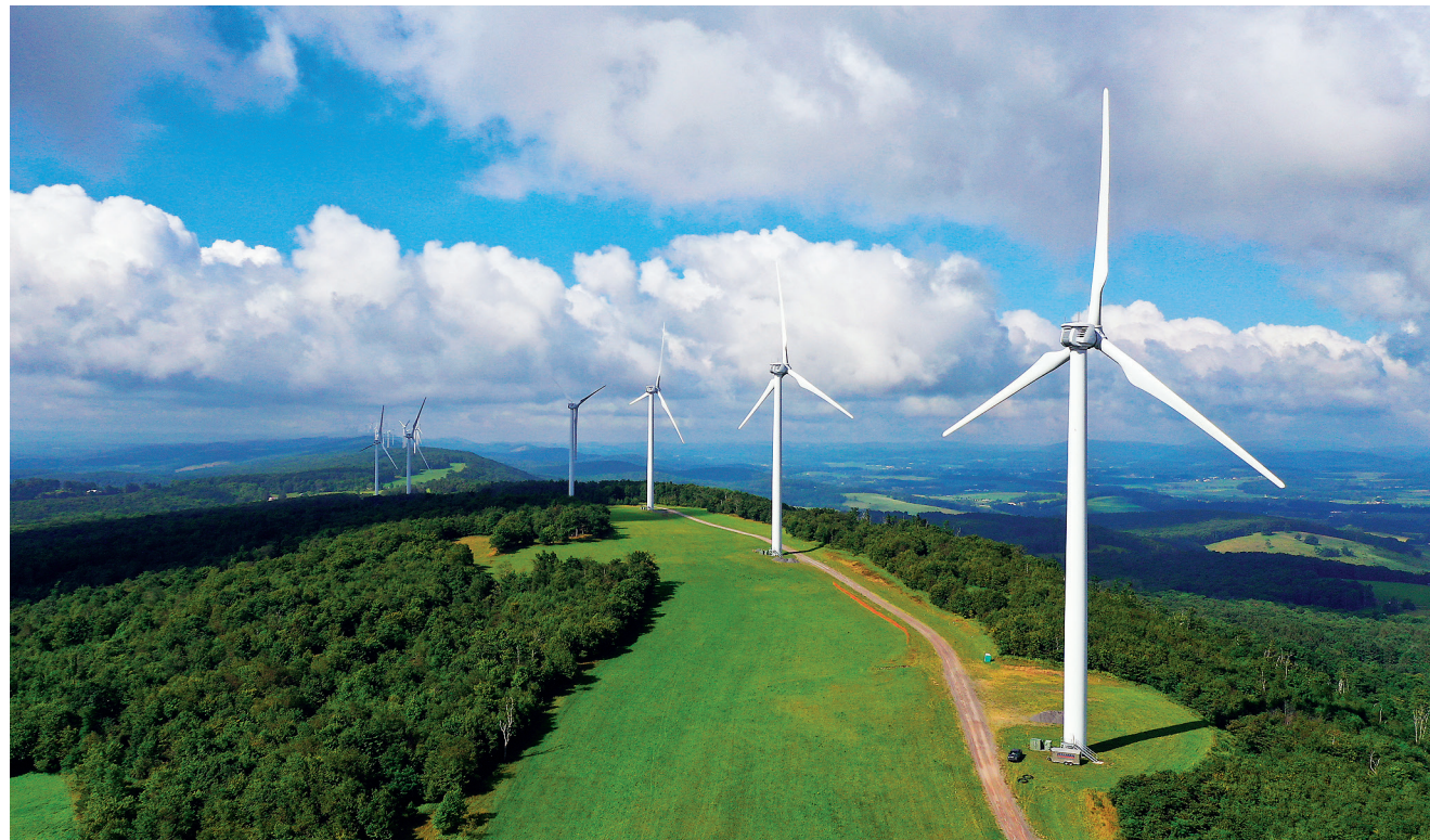
Turbines of Constellation Energy's Criterion Wind Project stand along the ridge of Backbone Mountain near Oakland, Md., on Aug. 23.
