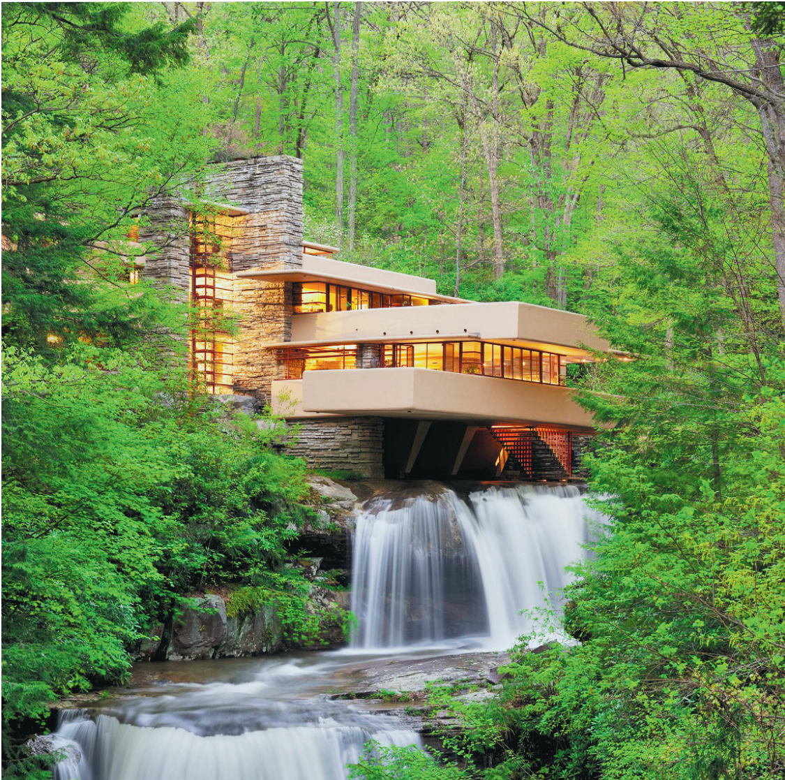
▲ Frank Lloyd Wright’s distinctive and daring cantilever design over a waterfall, using reinforced concrete, achieved not only a unique modern aesthetic but also safety over the falling water.
