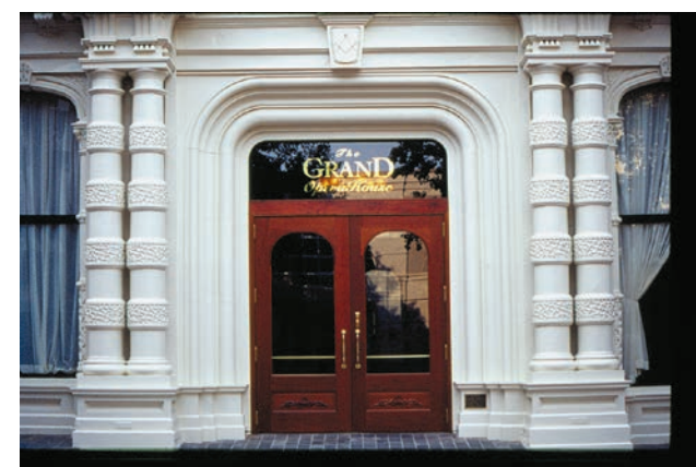
▲ The main entryway of the Grand Opera House evokes a bygone era with decorative solid wood doors featuring its name etched into the glass, as well as highly distinct, painted cast-iron double columns.
