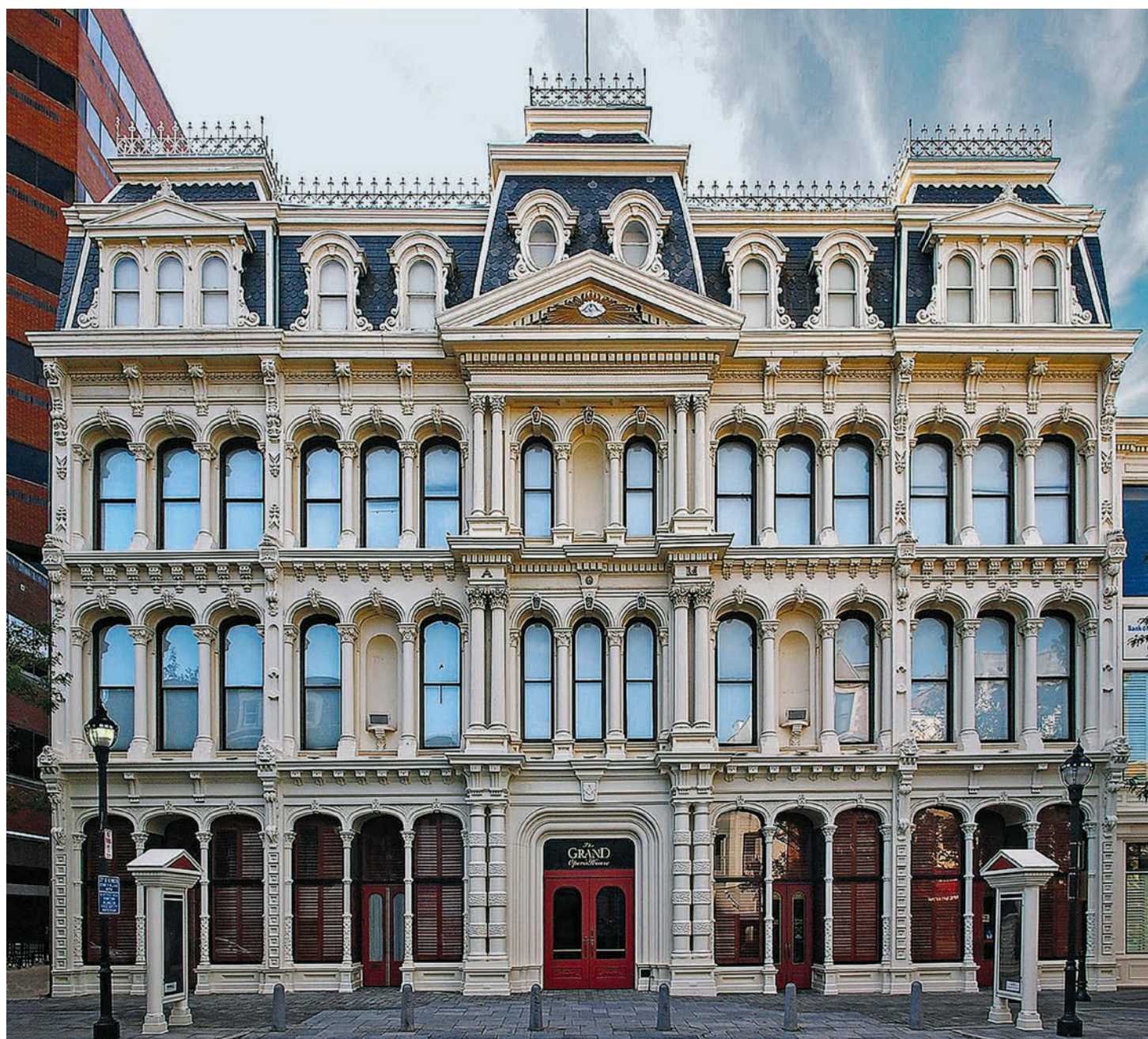
▲ Famed 19th-century architect Thomas Dixon was inspired by the design of the Paris Opera House, which shows off a French Second Empire style, an eclectic compilation of different architectural elements from various time periods. At 92 feet, the façade impresses with its various arches, Masonic symbols—especially the eye of providence—as well as Corinthian columns, dental molding, and much more.
