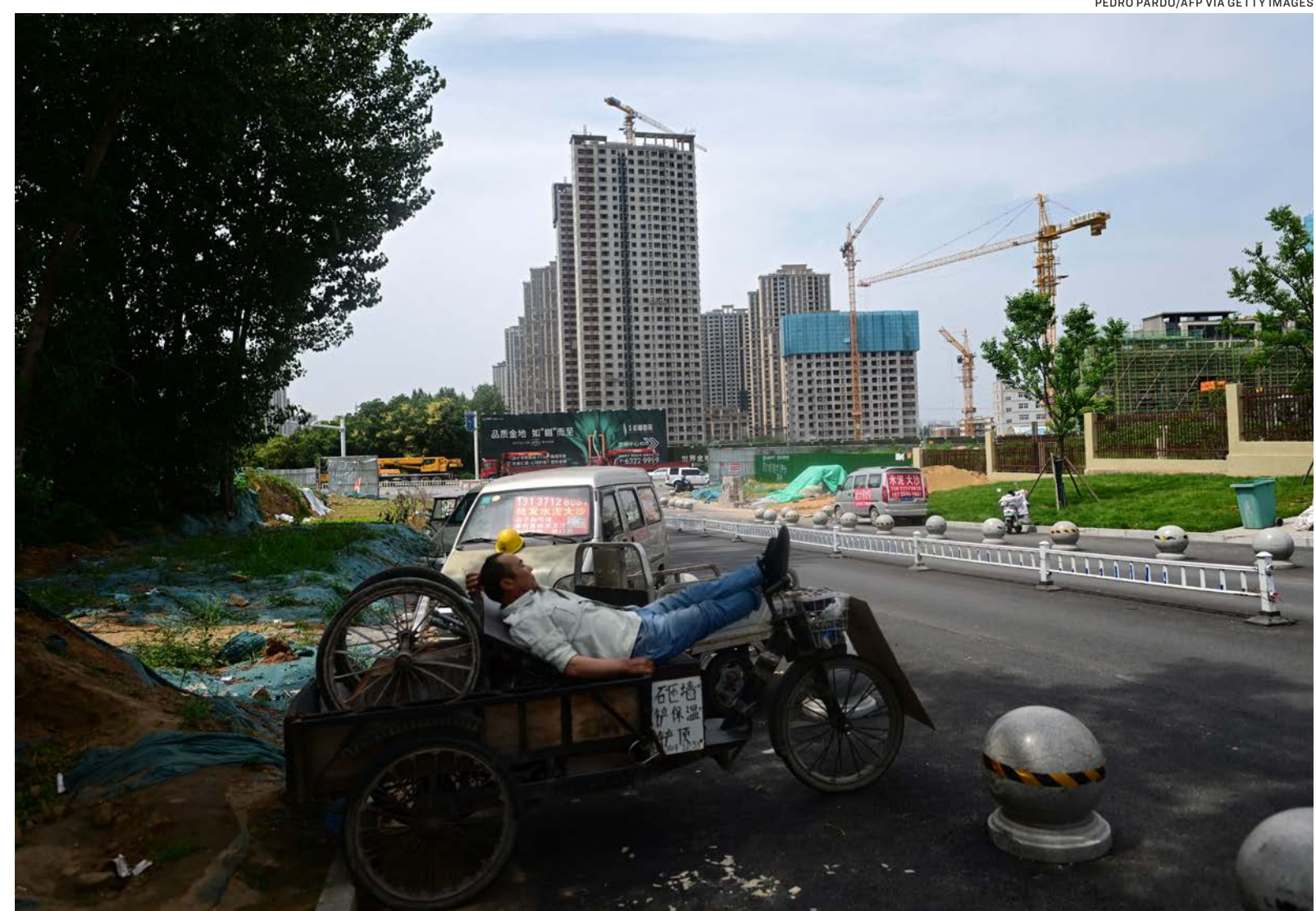
▲ A man rests in front of a housing complex under construction in Xinzheng, Henan Province, China, on June 20, 2023.
