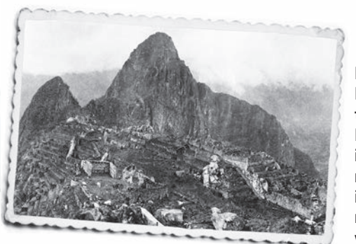
Photograph of Machu Picchu taken by Hiram Bingham III in 1912 after major clearing and before reconstruction work began.
