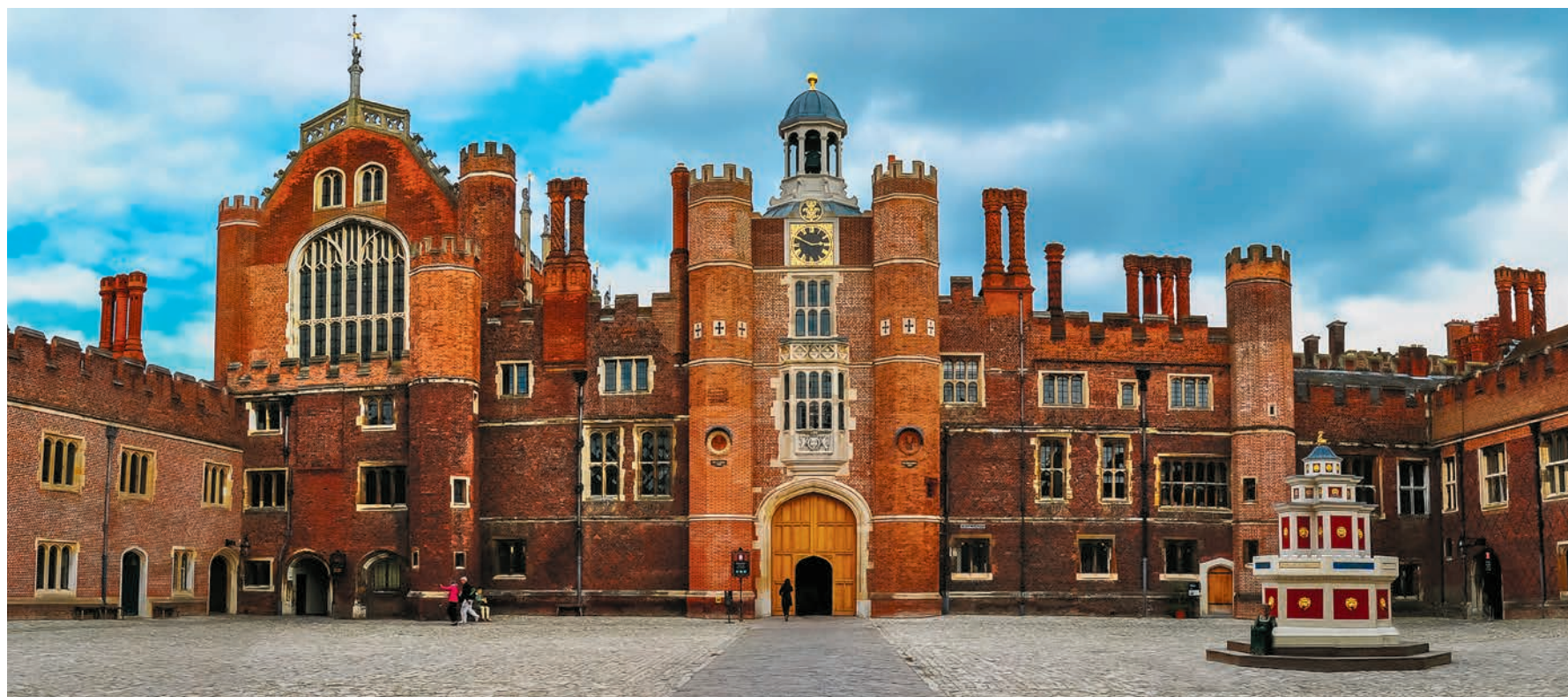
▲ The west façade of Hampton Court was built in the Tudor style with its red brick, rows of rectangular windows, set of chimneys, and elaborate rooftops featuring gables. The façade features handmade bricks, tiles, stone, timber, and lead. Vitrified bricks form the large crisscross pattern that decorates the palace courtyard. At the center of the building is Anne Boleyn’s gatehouse, with an elaborate octagonal Tudor wine fountain on the right.
