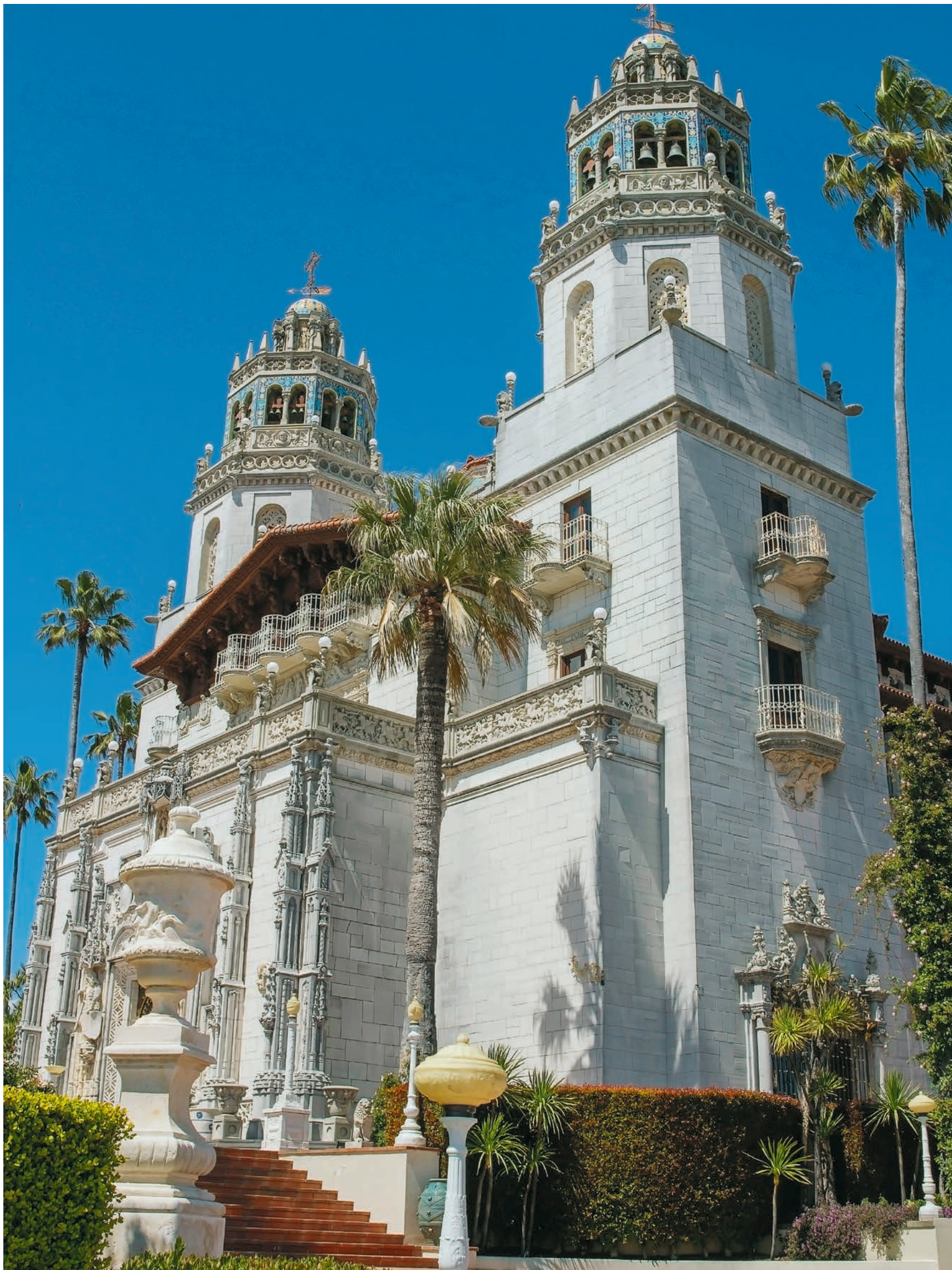
Architect Julia Morgan is best known for her work on the Hearst Castle. Front view of the castle in San Simeon, Calif.
