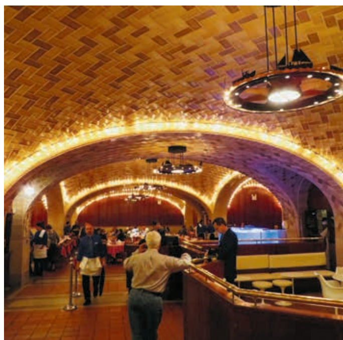
Guastavino's tiles cover the ceiling of the Grand Central Oyster Bar &amp; Restaurant in Manhattan, N.Y.
