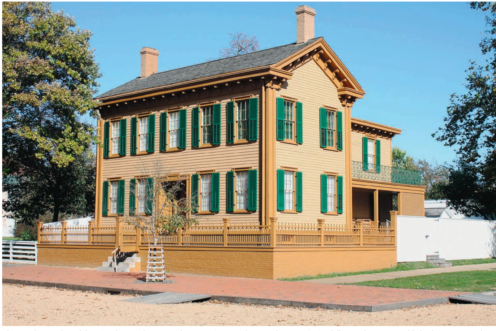
The Lincolns purchased their Greek Revival one-story home in 1844. Twelve years later, in 1856, a full second story was added to become a nearly 3,000-square-foot home. Renovations included Italianate details, such as a low-pitched roof and projecting eaves with large brackets.
