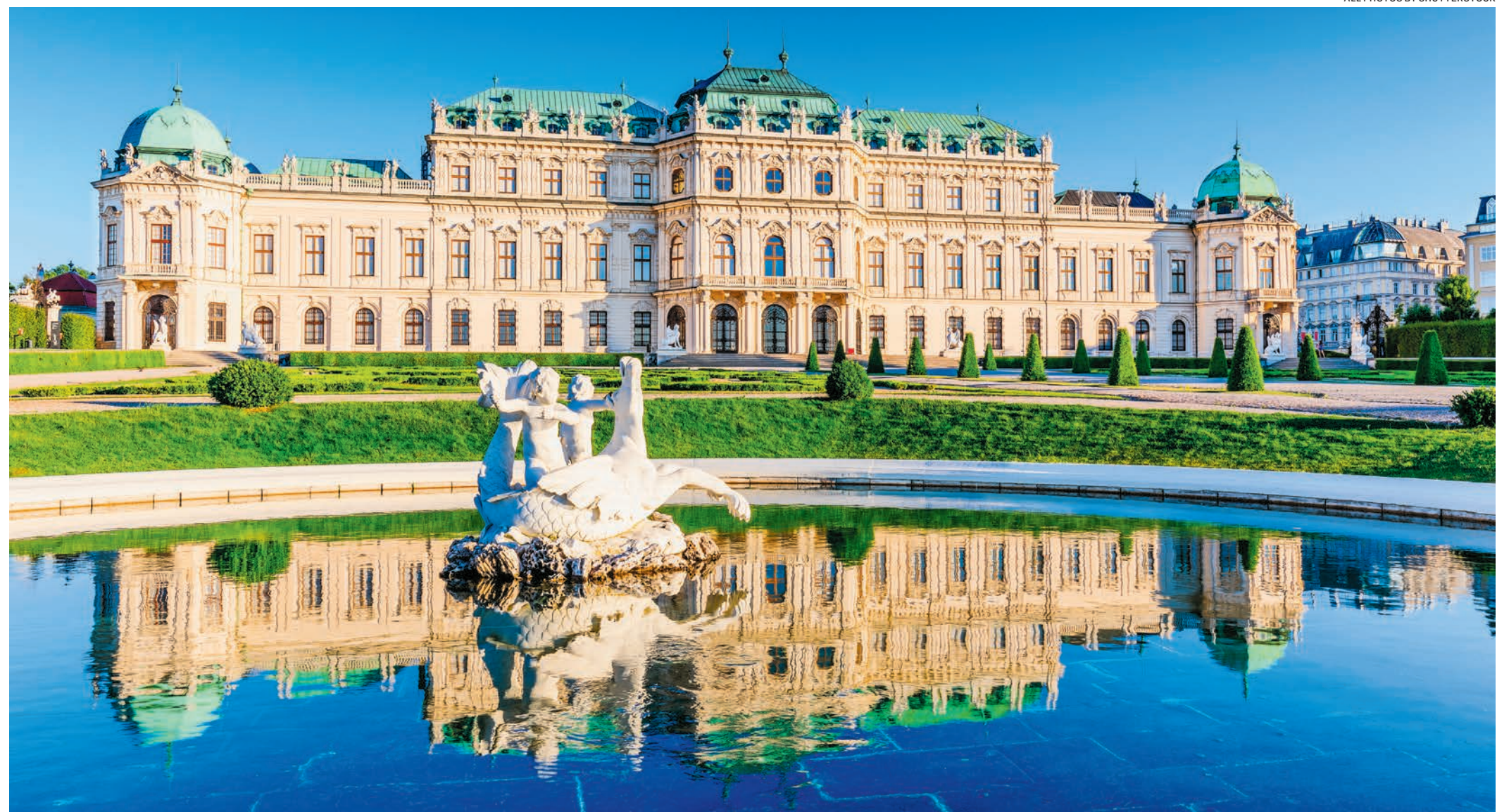
The Upper Belvedere palace in the center of Vienna, Austria. The building is composed of a long range of 29 bays, articulated as seven octagonal pavilions, with ornamented pilasters and window surrounds. These pavilions are in a typical 18th-century French design, which can be seen in the Tuileries Garden in Paris or at the Palace of Versailles.
