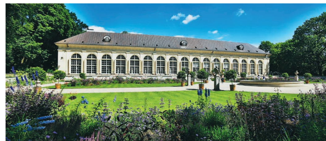
Italian-Polish architect Domenico Merlini worked at the king's court and designed the Old Orangery. Built between 1785 and 1788, the neoclassical building houses the Royal Sculpture Gallery and the Royal Court Theater, the present home of the Polish Royal Opera.
