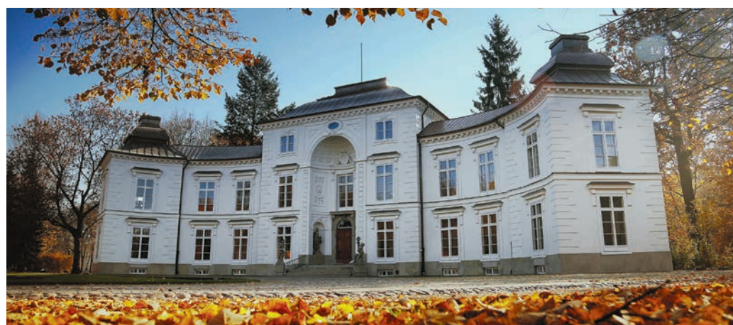
The apartments of King Stanislaw August's heir and nephew, Prince Jozef Poniatowski, can be found in the Myslewicki Palace. The semi-circular neoclassical palace is topped with curved copper roofs that reflect Chinese-style architecture. Visitors enter the palace through a tall niche flanked by statues of Flora and Zephyr.
