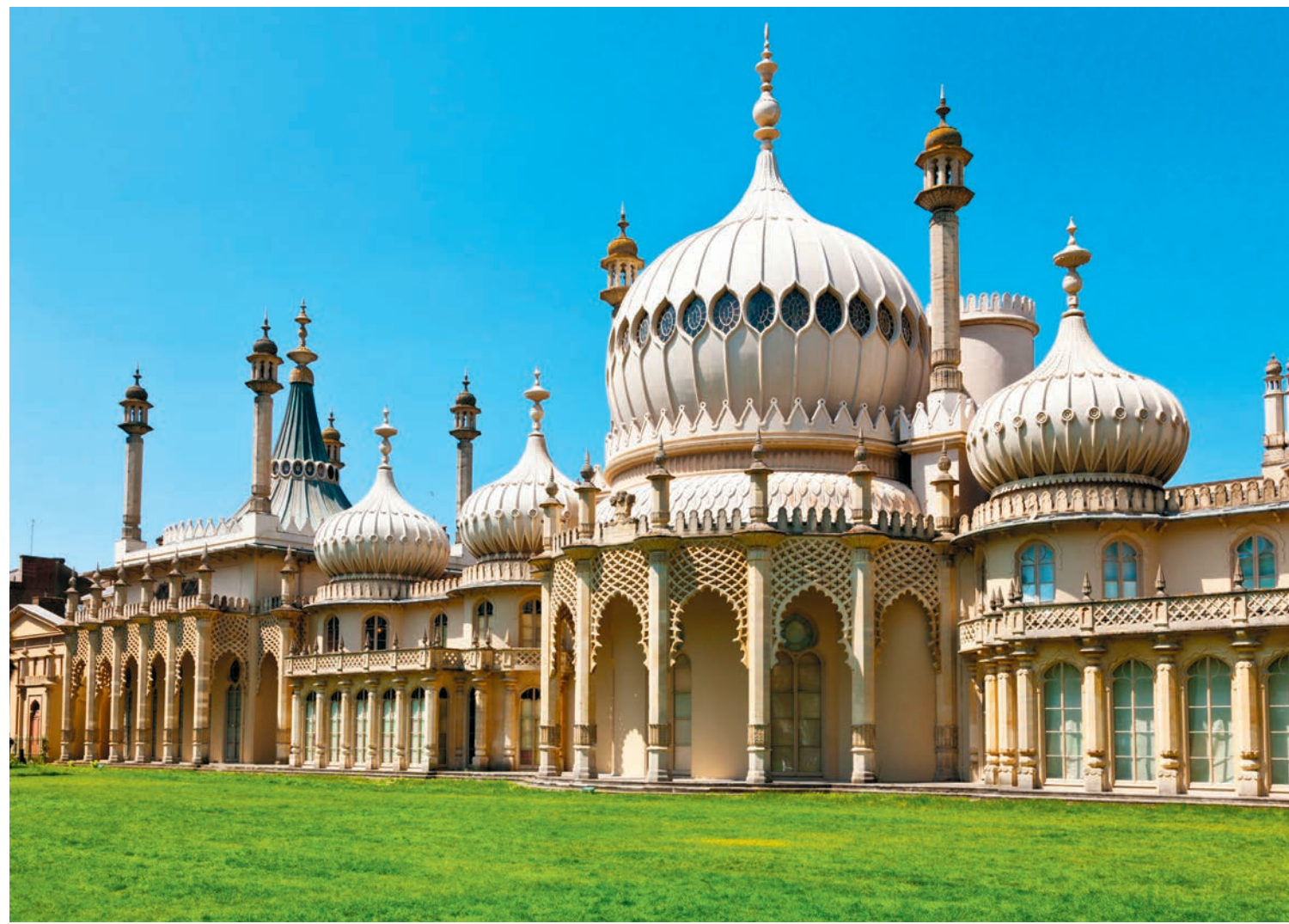
(Left) The exterior of the pavilion, featuring cast-iron onion domes, pinnacles, and pointed arches. Architect John Nash added an iron frame to architect Henry Holland's original construction to support 10 domes and 10 minarets, contributing to a unique Indo-Islamic appearance. Noticeable are the arabesques (surface decorations in Islamic architecture), columns, and ornate arched windows.
