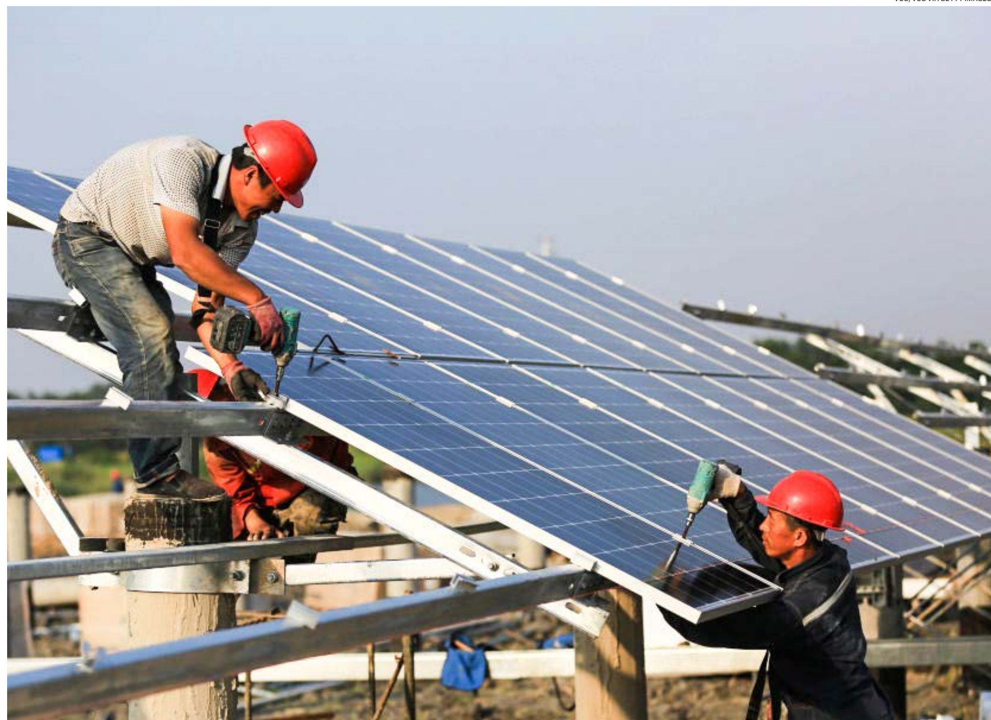
Workers install solar panels at the construction site of 40MW photovoltaic on-grid power project in Huai an, China, on June 11, 2018.
