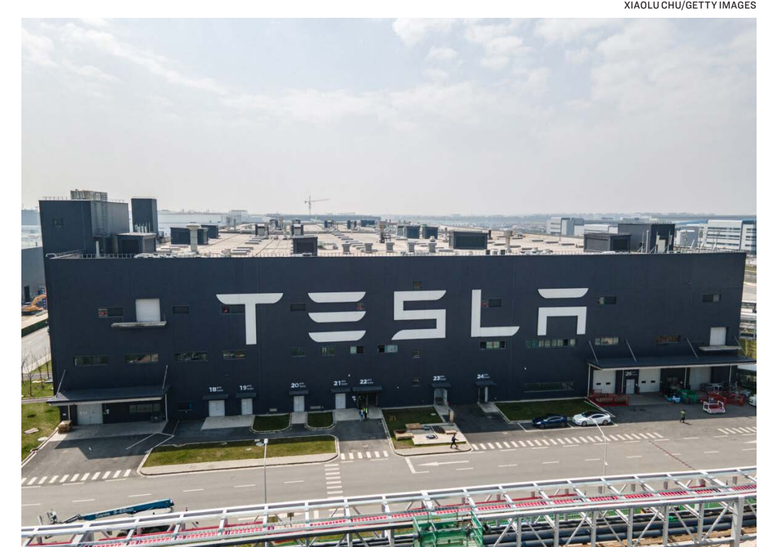
The Tesla Shanghai Gigafactory in Shanghai on March 29, 2021.
