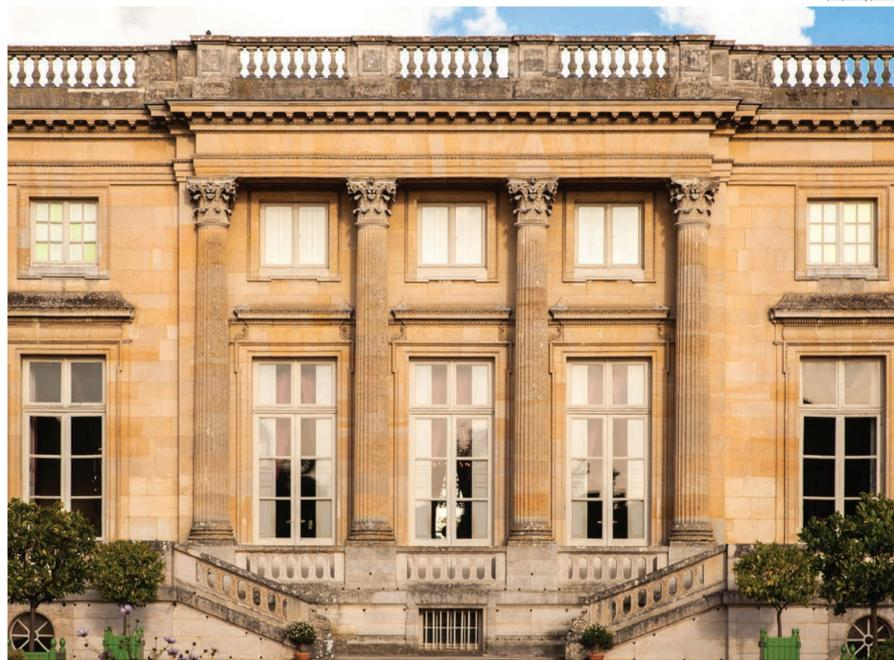
The main façade of the Petit Trianon. The structure has a balustrade atop the roof that softens the edge of the building and extends the vertical lines established by the Corinthian columns.
