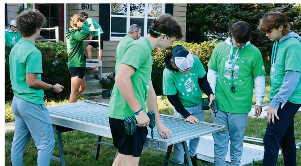
Students from Badin High School at work on the wheelchair ramp.
