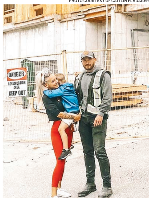
Noah Fladager with his wife Caitlin and son in front of a new hotel where his company has been contracted to do some plumbing work.
