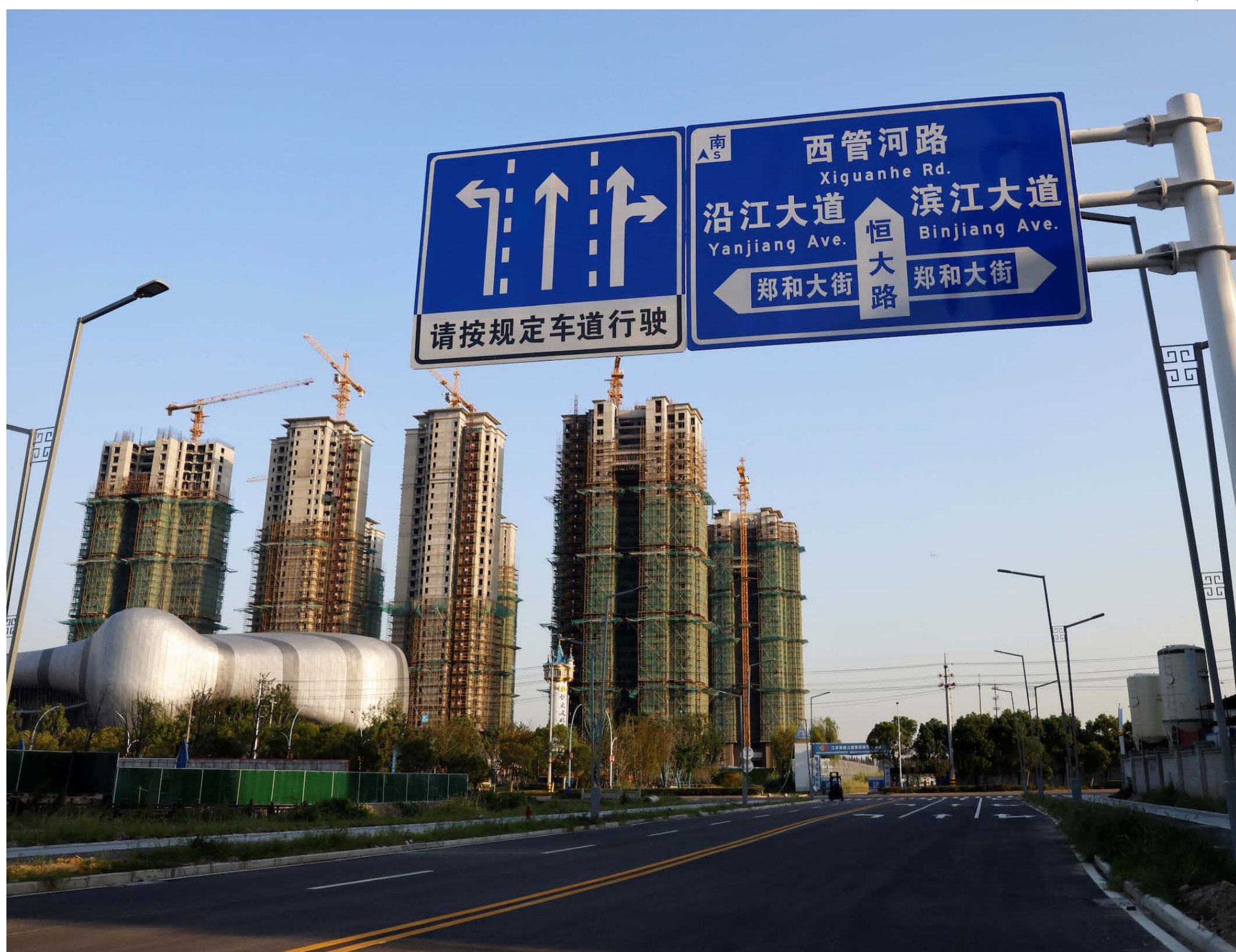
Residential buildings under construction are seen at a project developed by China Evergrande Group, in Suzhou, Jiangsu Province, China, on Sept. 23, 2021.
