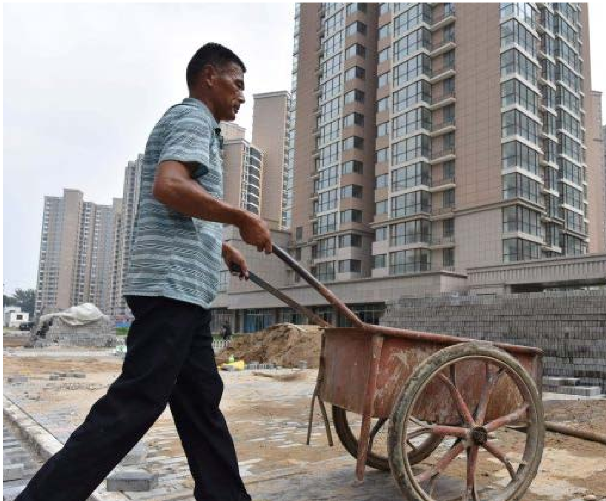
A worker pushes cart at the construction site of a housing complex under construction in Beijing on Aug. 15, 2017.
