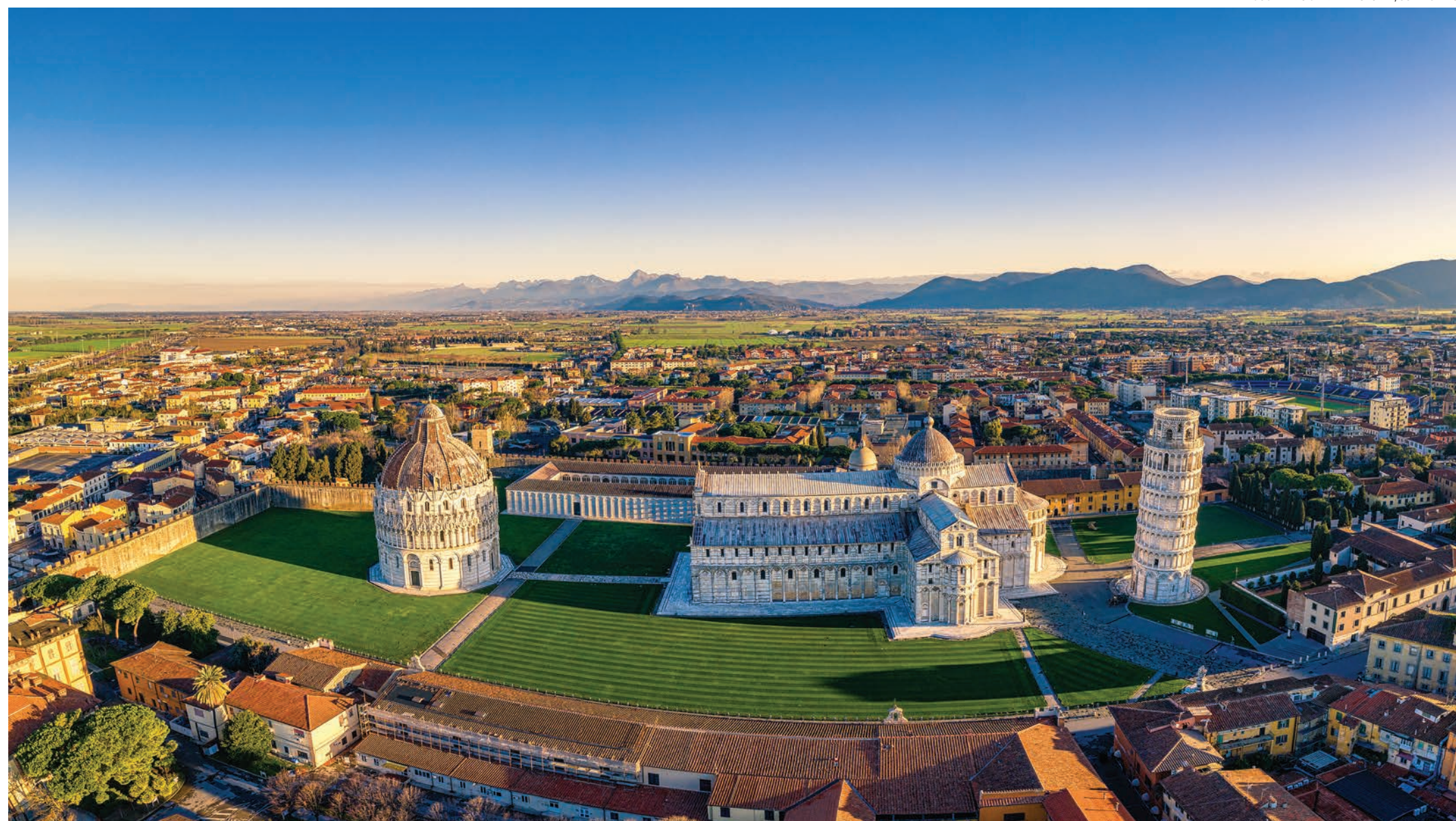
(Above) The monuments stand on display in the early morning light, serving the people of Pisa and the heavens above. (Below) Made from white marble, the tower is estimated to weigh almost 16,000 tons. Upon completion of construction in 1319, the tower tilted 1 degree. It has leaned as much as 5.5 degrees but currently stands at an approximate 4-degree tilt after a restoration effort.
