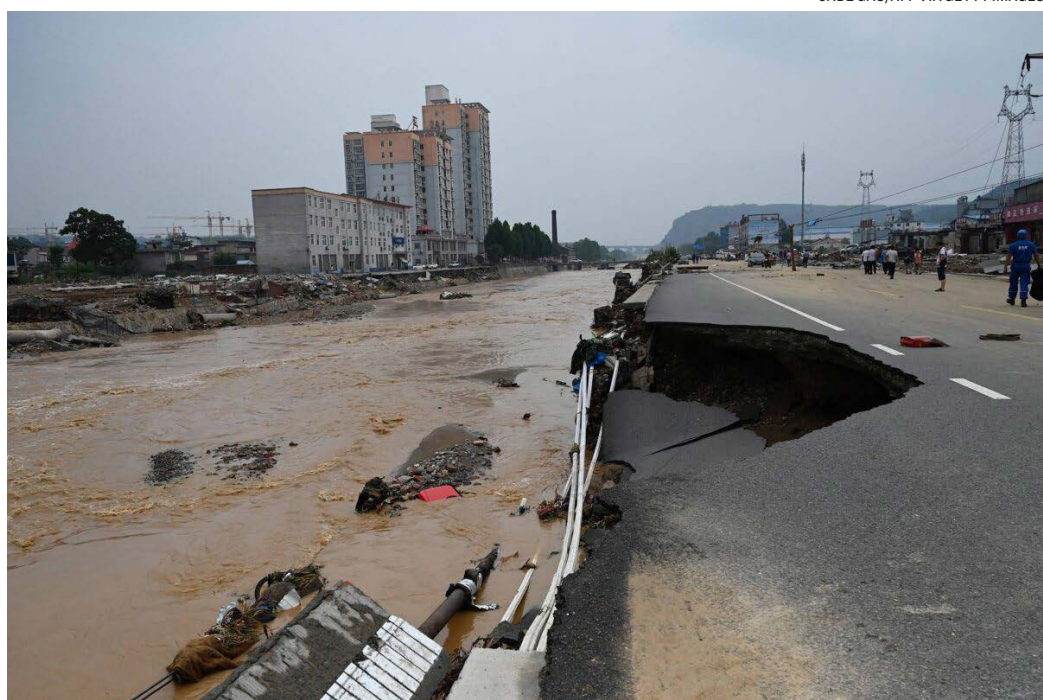
A road collapses after severe flooding and landslides in recent days have hit the county-level city of Gongyi, near Zhengzhou, in central China's Henan Province on July 22, 2021.
