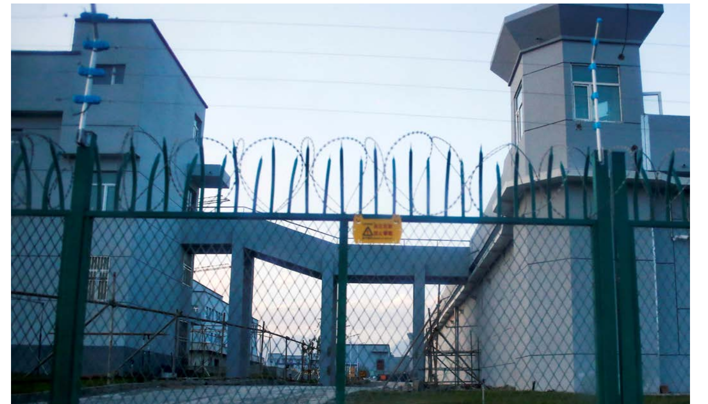
A perimeter fence is constructed around what is officially known as a vocational skills education center in Dabancheng in Xinjiang Uyghur Region, China, on Sept. 4, 2018.
