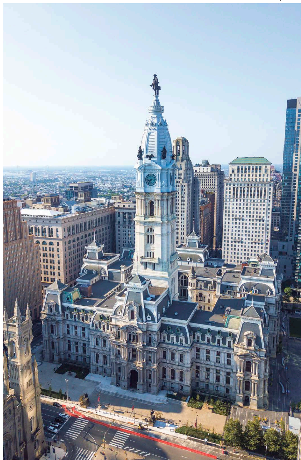
(Above left) The building's form is quadrangular, with a large courtyard and turrets at each corner. The convex-curved Mansard roof, made of slate, with large dormer windows, defines the building in a distinctive French style. (Above middle) This portal stairwell is made of limestone walls, with granite for the steps, columns, and base, and limestone for the heavy carved railings. The stairwell provides access to the upper levels while allowing natural light to penetrate deep into the building. (Above right) One of the staircases in the north and south portals. The grand scale is felt upon looking up at the coffered ceiling, seven stories above the ground.
