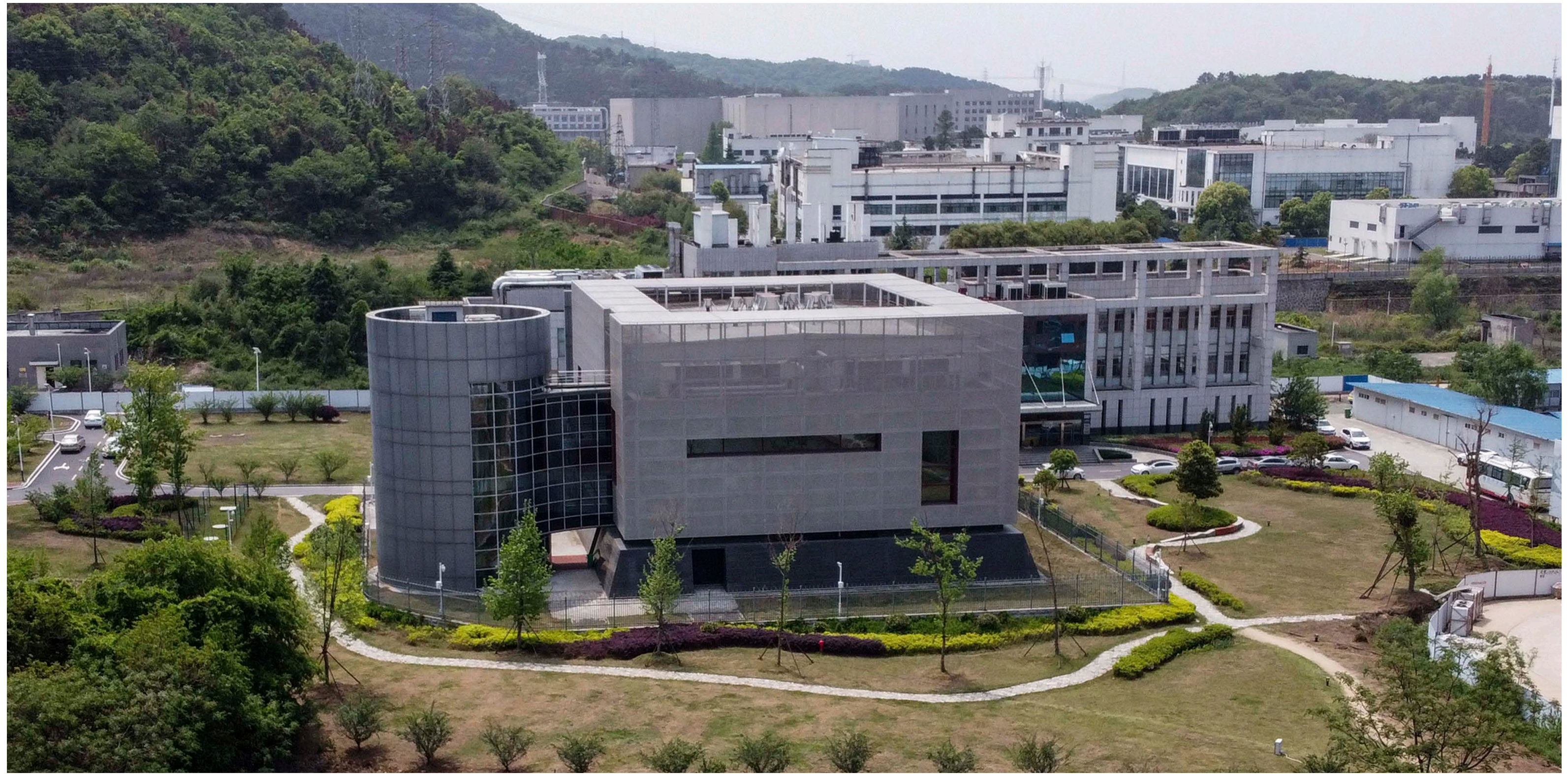
↑ An aerial view of the P4 laboratory at the Wuhan Institute of Virology in Wuhan, China, on April 17, 2020.
