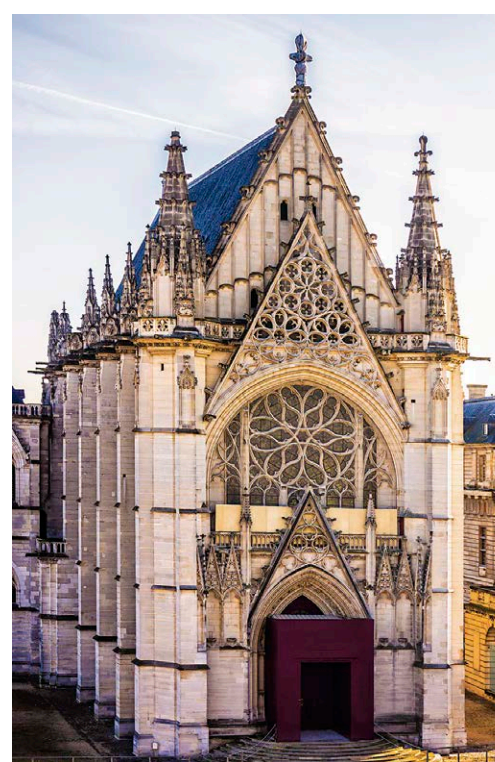
(Left) The distinctive narrow buttresses of Sainte-Chapelle take on the bulk of the weight-bearing so that the stained glass can stay upright. (Right) The entrance to Sainte-Chapelle.
