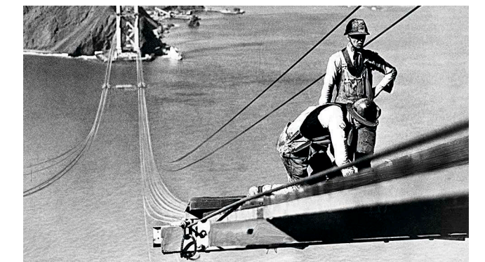
Men at work on the construction of the Golden Gate Bridge in San Francisco in this file photo.
