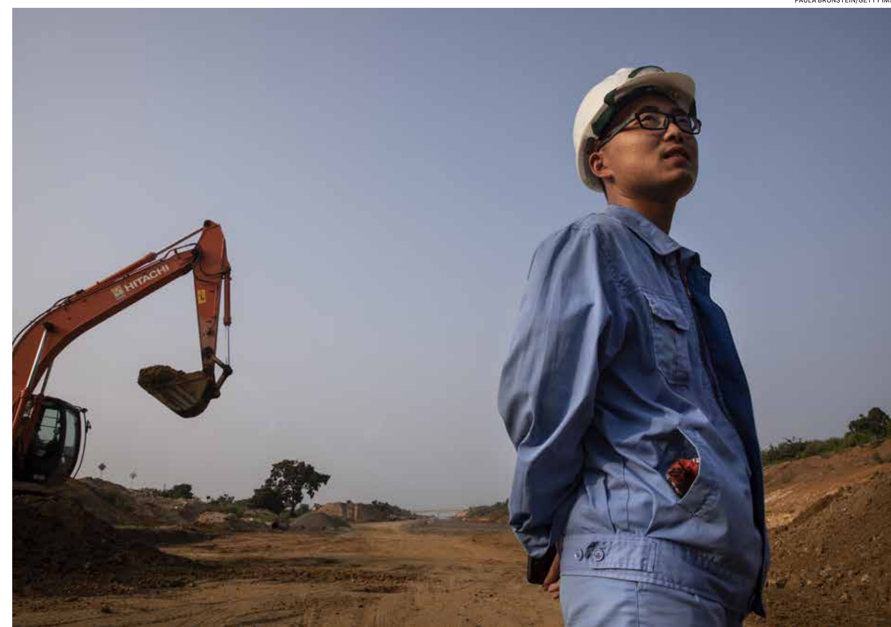
A Chinese engineer at the construction site of an extension of the Southern Expressway from Matara to Hambantota, near Hambantota, Sri Lanka, on Nov. 16, 2018.
