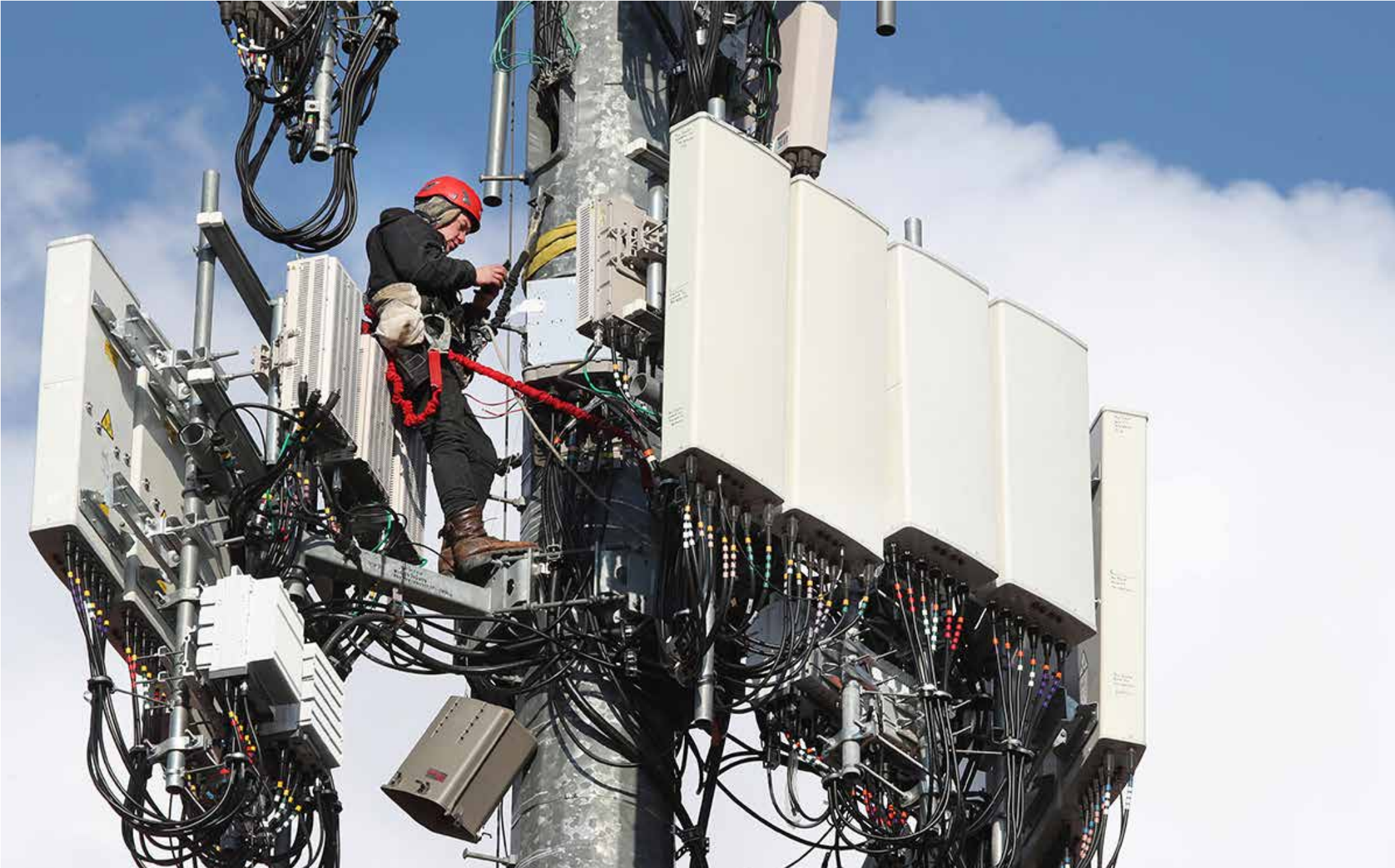
A worker rebuilds a cellular tower with 5G equipment for the Verizon network in Orem, Utah, on Nov. 26, 2019.
