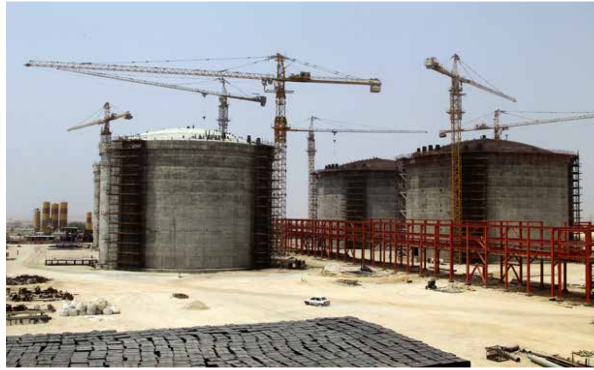
South Pars gas field development in the southern Iranian port town of Asaluyeh, in this file photo.
