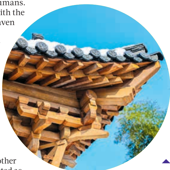
Dougong or interlocking brackets are a feature of traditional Chinese building that relied on wood.
